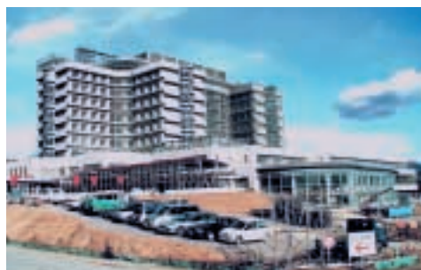
Shizuoka Cancer Center Electric works for Hospital Bldg.
