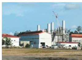
Combined cycle power generation station (Dar Salaam, Brunei)
