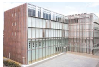
Kyoto headquarters of Nissha Printing Co., Ltd.
