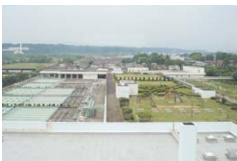
Tamagawa Upstream Water Recycling Center of Tokyo Metropolitan Waterworks Bureau
