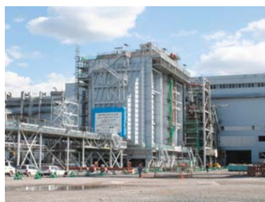
The Tokyo Electric Power Company's Futtsu Thermal Power Station
