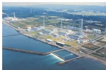
Kashiwazaki-Kariwa Nuclear Power Station (courtesy of The Tokyo Electric Power Company, Inc.)
