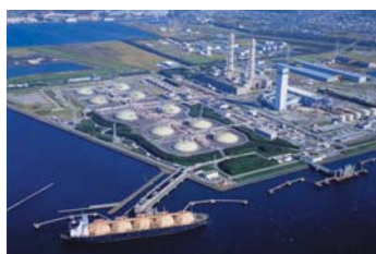
The Tokyo Electric Power Company's Futtsu Thermal Power Station (courtesy of The Tokyo Electric Power Company, Inc.)
