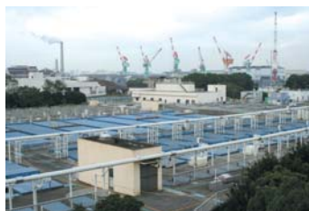
Yokohama City Government Bureau of Sewerage North No. 2 Water Recycling Center
