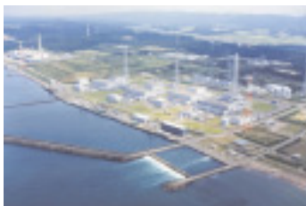
Kashiwazaki-Kariwa Nuclear Power Station (courtesy of The Tokyo Electric Power Company, Inc.)
