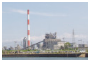
Mikawa Power Plant, Sigma Power Ariake Co. Ltd.
