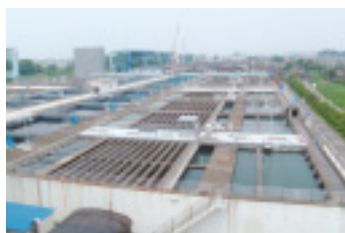
Samukawa No. 3 Purification Plant, Kanagawa Prefectural Public Enterprises Agency
