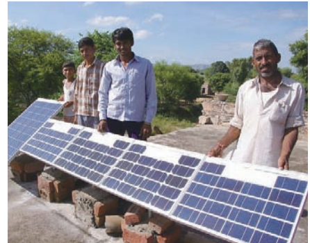
Station to charge solar lanterns using sunlight
