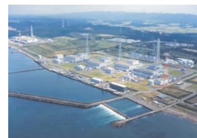
Kashiwazaki-Kariwa Nuclear Power Station (courtesy of The Tokyo Electric Power Company, Inc.)
