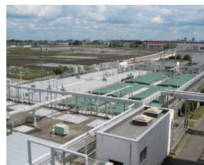
Shingashigawa upstream water circulation center, Saitama Sewage Corporation
