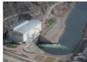
Nam Ngum 2 Hydroelectric Power Station, Lao People's Democratic Republic
