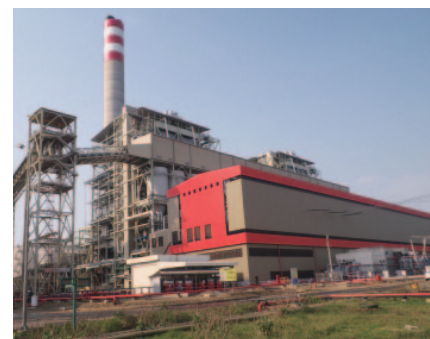
Tanjung Jati Power Plant, Republic of Indonesia
