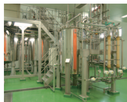
Construction of a new food plant (construction and facilities)
