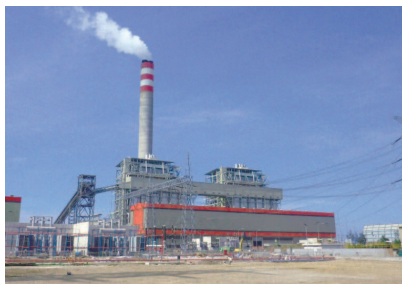
Tanjung Jati B Power Plant
