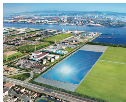
Fukuyama Solar Power Plant, The Chugoku Electric Power Co., Inc.
