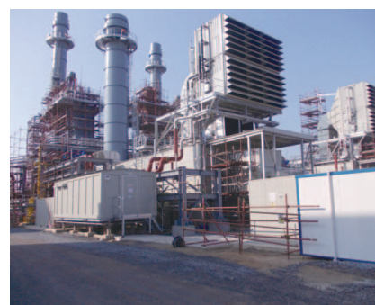
Amata Nakhon Power Plant, Thailand
