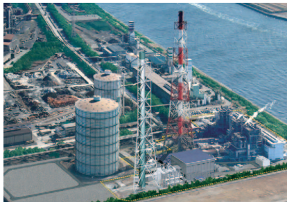
Image of completed No.4 unit of JFE Steel Corporation Chiba Works West Power Plant
