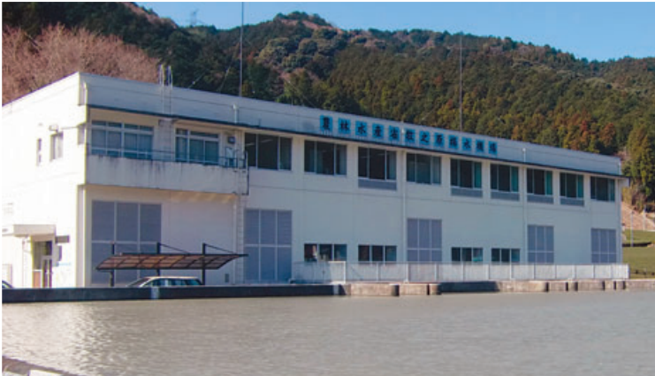
Kanto Regional Agricultural Administration Office Makinohara Irrigation Pumping Station
