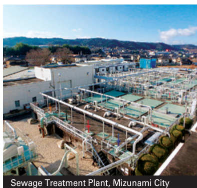
Sewage Treatment Plant, Mizunami City
