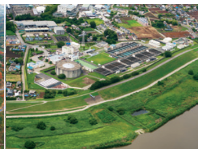
Showa Water Purification Plant (Saitama Prefecture Bureau of Public Enterprise)
