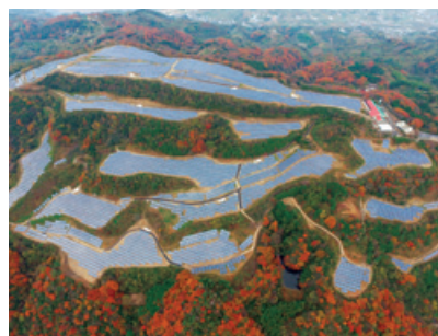
Sun-Earth Kinokawa No. 1 and No. 2 Solar Power Plants
