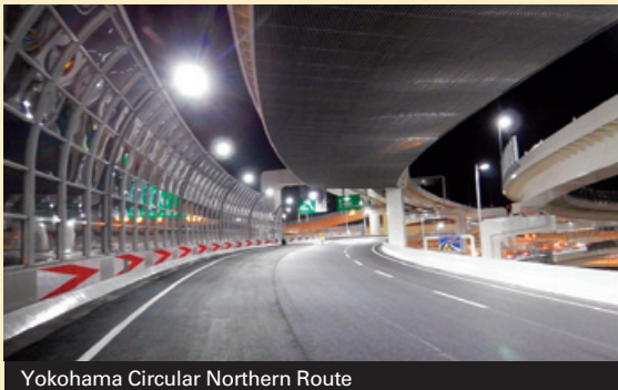
Yokohama Circular Northern Route
