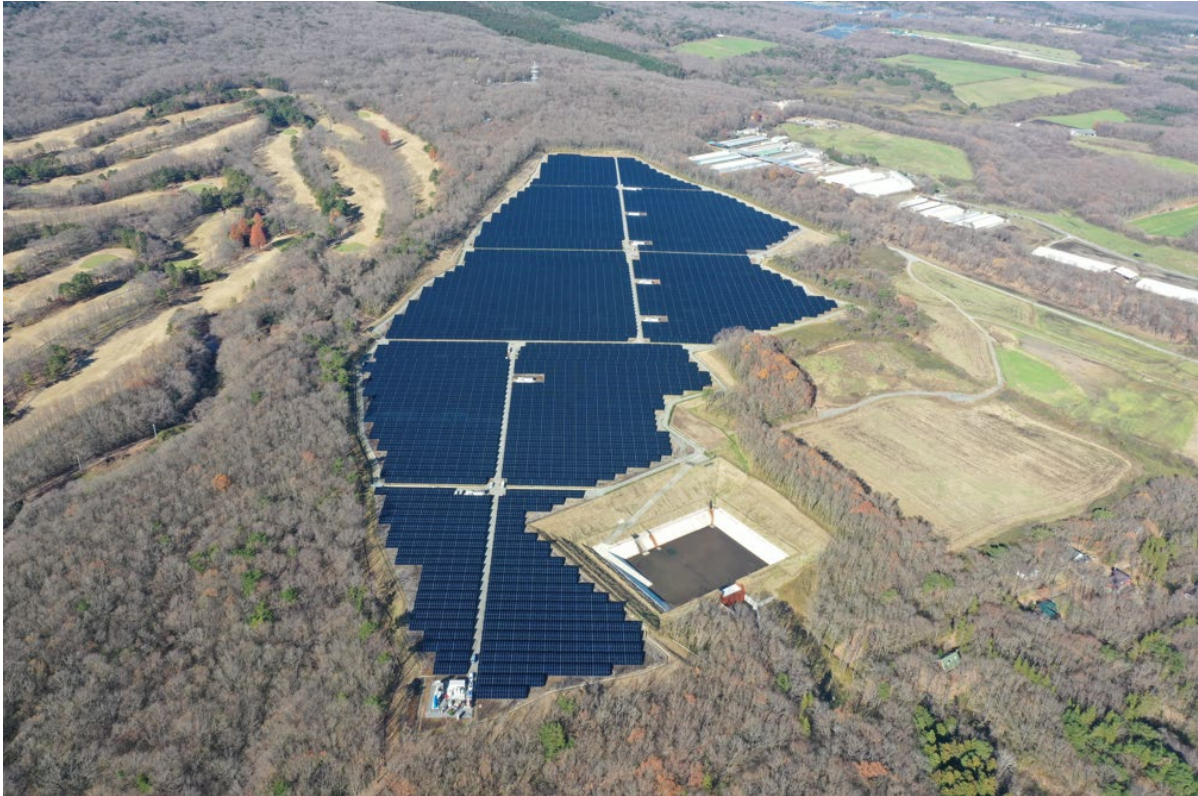
Mega-Solar Power Plant of PAG Renewables
